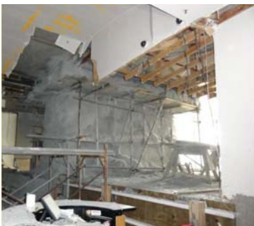
Overall View of Repair Using Shotcrete
