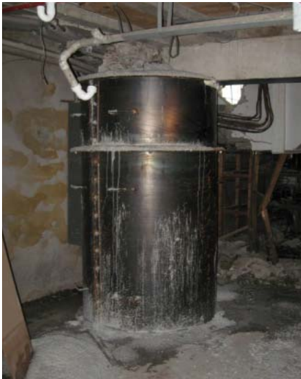
Damaged columns with completed encasement
