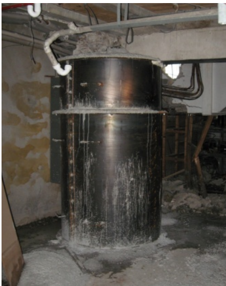
Damaged columns with completed encasement 4-9
