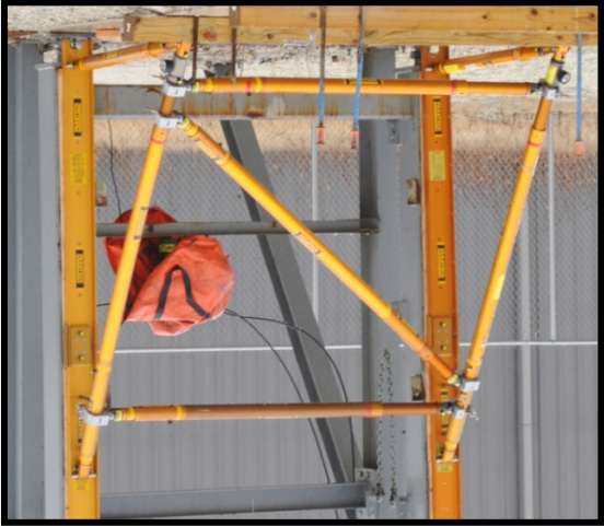
Photo using raker strut
