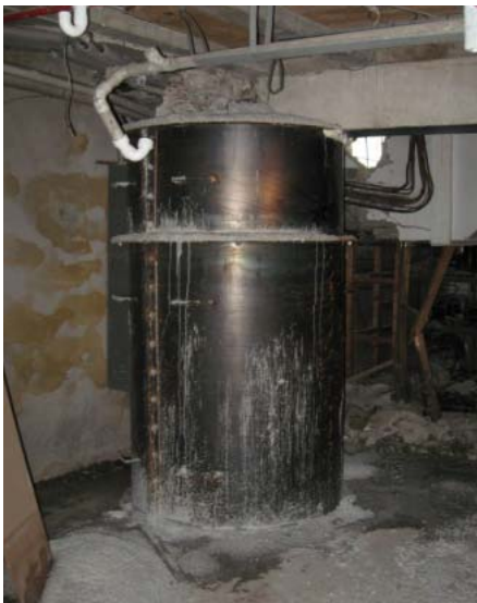
Damaged columns with completed encasement
