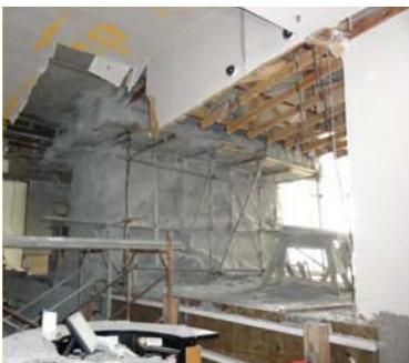
Overall View of Repair Using Shotcrete
